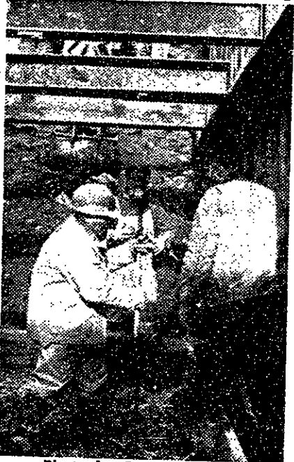
— Photo by Conrad Grundlehner Workmen prepare molds for a concrete base to contain two pipes carrying cooling water to the Magnet Laboratory.
