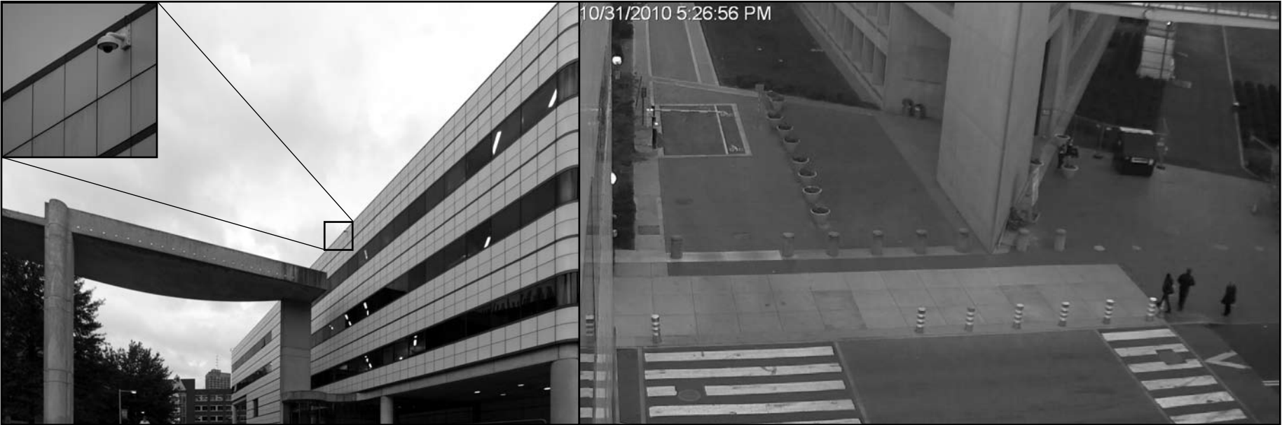
A security camera overlooks the vehicle entrances to campus on both sides of Bldg. 66; it was installed in early September. Left: The camera is mounted on Building E15, the old Media Lab building ( inset: detail on the camera). Right: Still frame from the security camera. It includes the gate to McDermott Court between the East Campus dormitory and Bldg. 66, and the driveway to the new courtyard in front of Bldg. 76, the Koch Institute.
