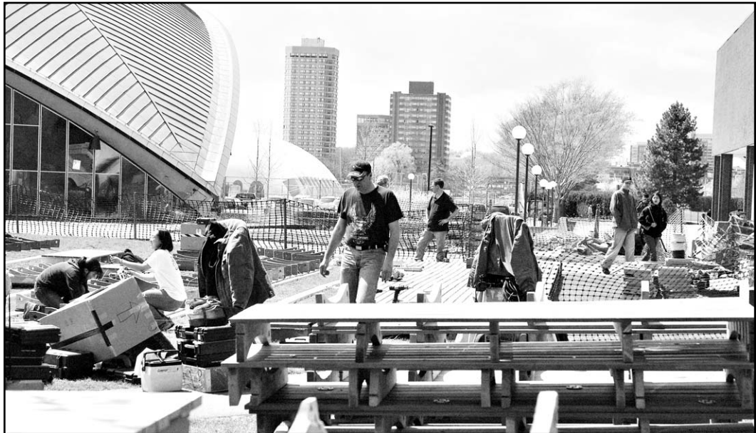
A group installs the interactive "White Noise/White Light" display for the inauguration of President Susan Hockfield, set to take place next Friday, May 6. The display, created by professor J. Meejin Yoon, will open in Kresge Oval this coming Monday, May 2.
