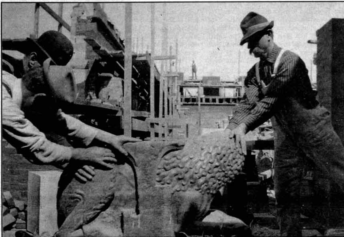
The Isabella Stewart Gardner Museum, under construction circa 1900.
