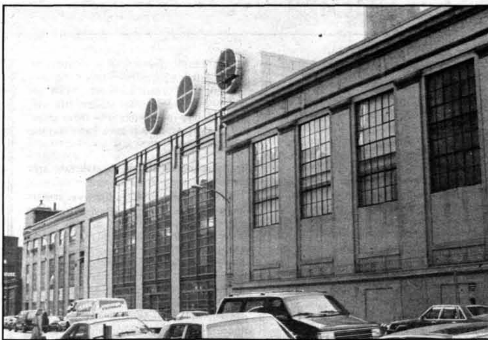
The $37 million new co-generation plant on Vassar Street opened Sept. 11.
