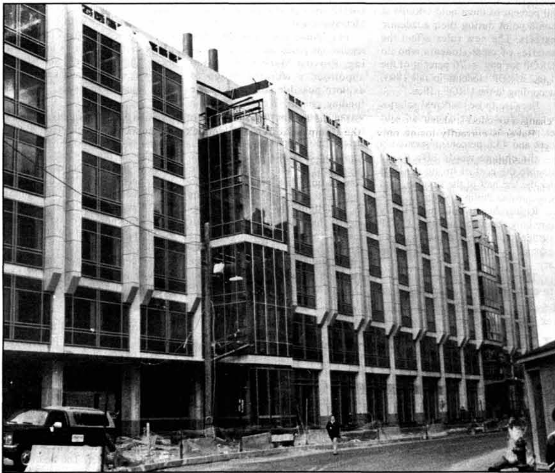
Building 68, the new biology building, nears completion last fall.
