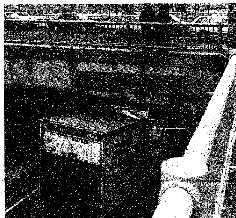
Prabhat Mehta/The Tech Bridge 1, truck 0. A truck slammed into the Massachusetts Avenue overpass Sunday evening, leaving behind its trailer.
