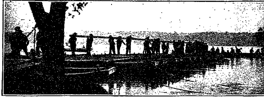
A Variety of Burdens Go to Make up a Ponton Bridge—Bridge building across Accotink Bay by the R. O. T. C. at Camp Humphreys last summer.
