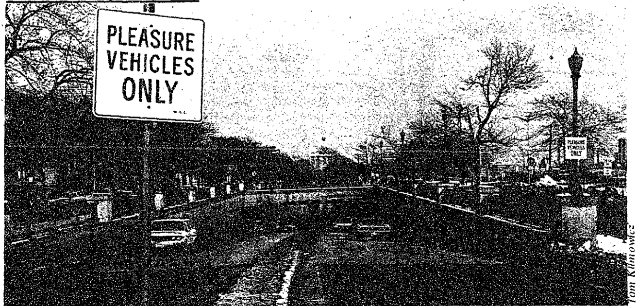
The nine foot underpass on Memorial Drive next to the Harvard Bridge has proved hazardous to truck drivers who ignore signs warning that trucks are not allowed on the drive. According to one estimate, about one truck crashes into the top of the underpass every week.
