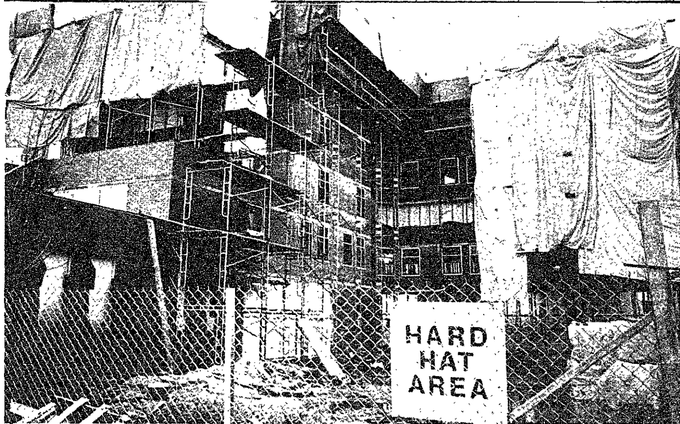
Work is progressing on schedule on the new west campus dorm. The only question mark now is the weather. Photo by Mark James
