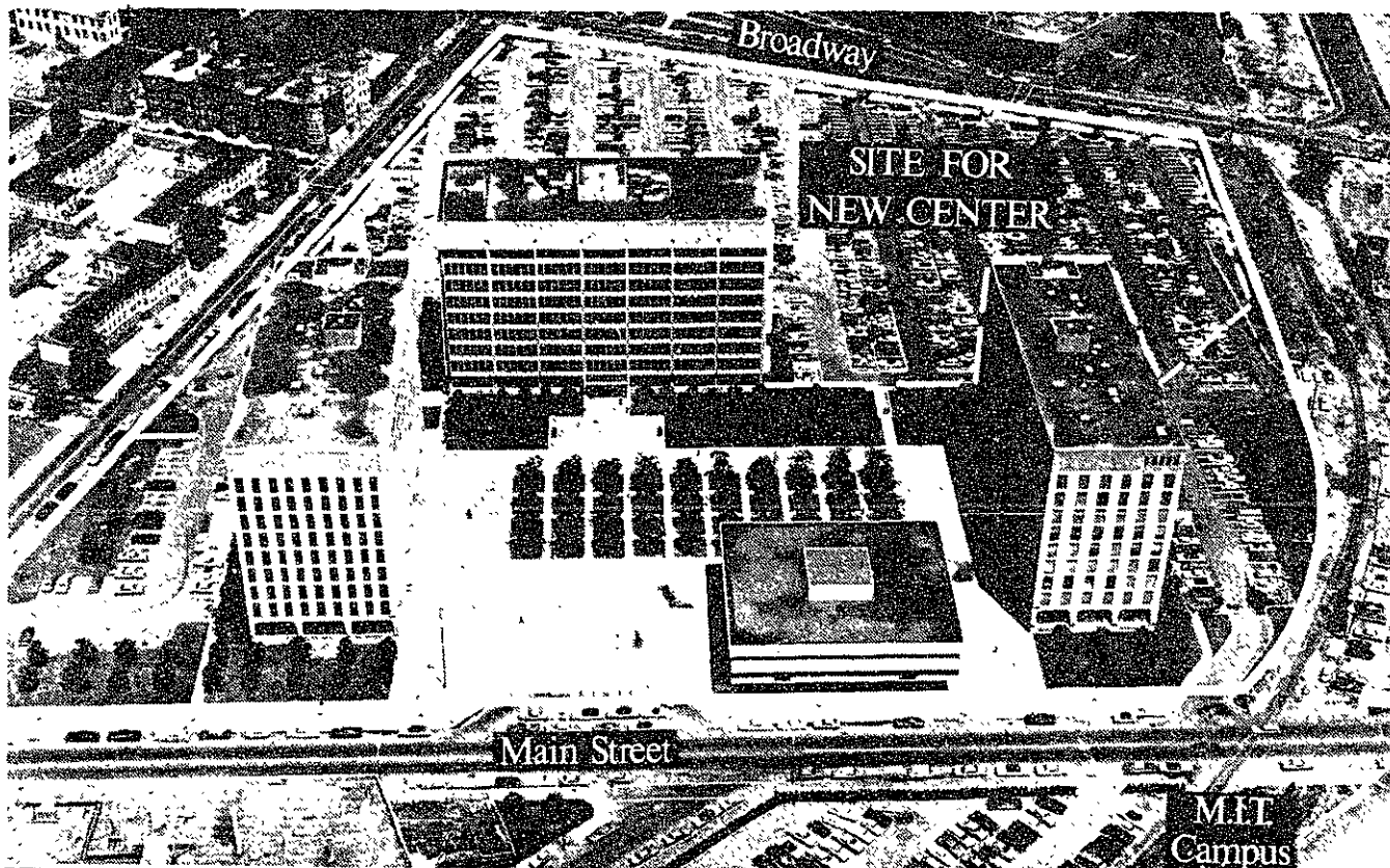
The new Tech Square location of the Charles Stark Draper Laboratories, Inc.
