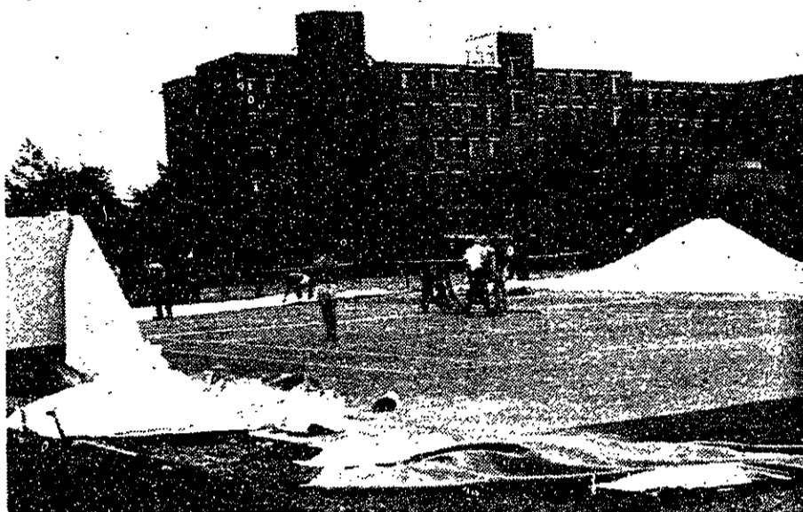
Above, aerodynamic stresses on a typical inflatable structure. High winds put undue stress on MIT's indoor tennis center, causing its downfall, below. Photo by David Searls
