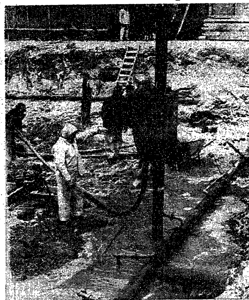
High pressure water is used to bore holes in the Earth Sciences construction site. Pipes sunk in these holes will be attached to the large horizontal pipe and will be used to drain the site of water when large-scale digging commences.
