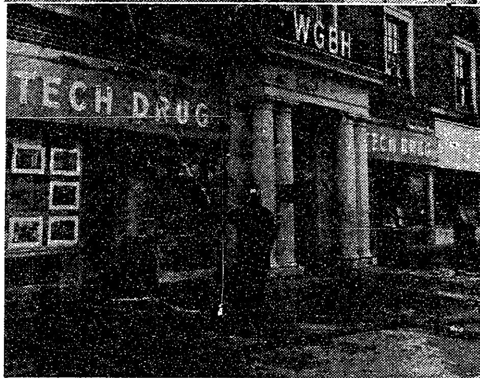
— Photos by Curtiss Wiler '63 A fireman seeks a spot to place some of WGBH's equipment carried out of the gutted building (top photo). Below, the front of the building late Saturday morning as the fire department made certain that the blaze had been fully extinguished.
