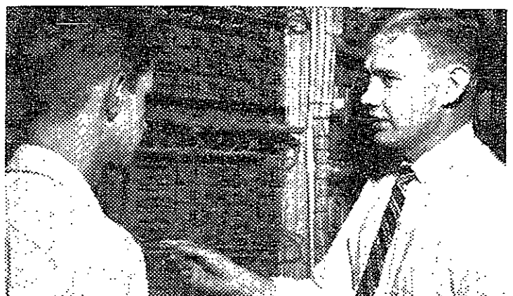
"10:45 a.m. Before any modifications can be made, it's important that I check apparatus and wiring options. That's what I'm doing here at the Remote Control Terminal equipment."
