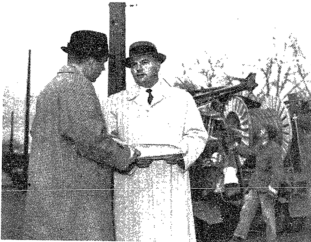
Ken Boekeloo (center foreground) at the scene of a cable installation project in Detroit.
