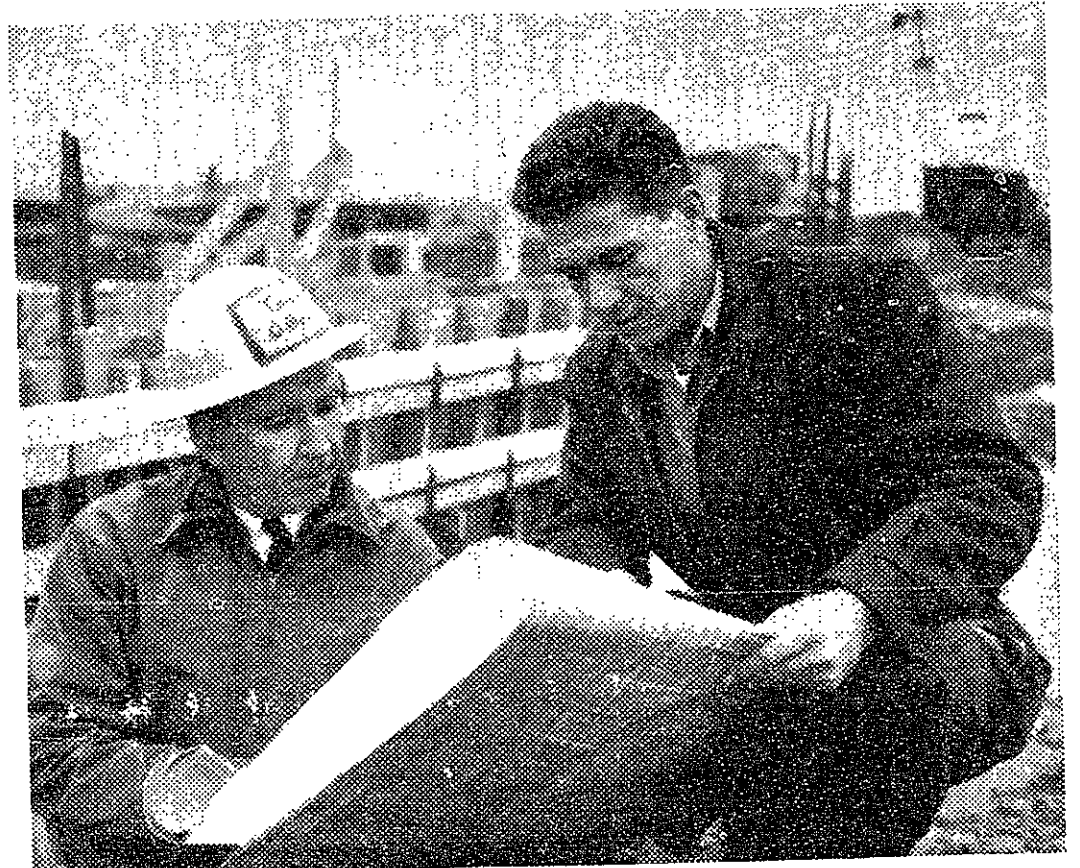
Cliff Downer (right), A.B. in Mathematics, '49, M.S. in Civil Engineering, '50, Harvard, on the site of a building construction project.
