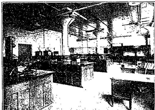
A Section of the SIMPLEX Electrical Laboratories
