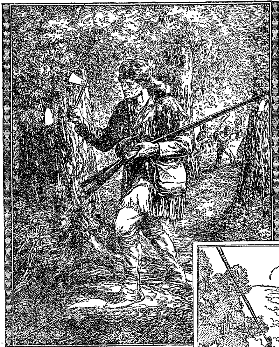
Today telephone cables cross country that Daniel Boone knew.
