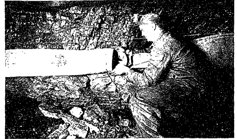
Coupling two VENTUBE sections
