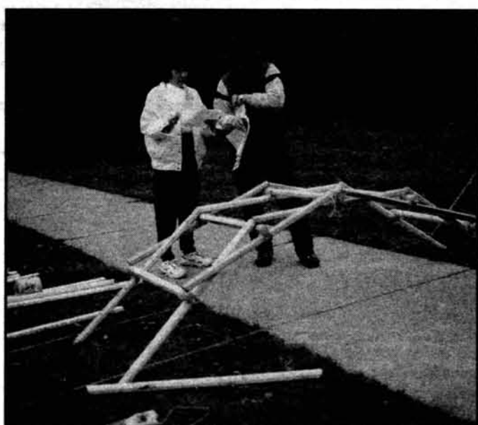
Marcus Brandt shows Deying Sun the plans for a Chinese Rainbow bridge that will be constructed near Singapore next month. Brandt, a member of the Traditional Timberframing Research and Advisory Group, is studying different methods of assembling and deploying the bridge.
