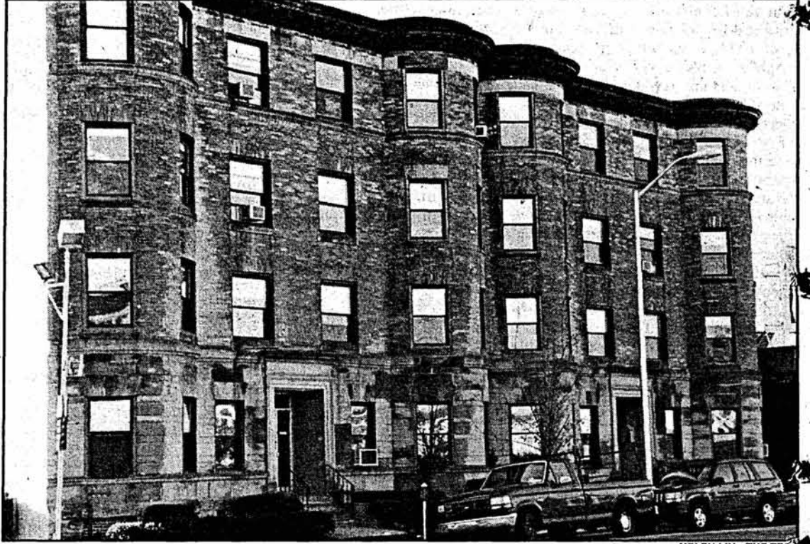
Repairs to Random Hall have largely undone the damage caused by blocked heating and sewage systems. Two weeks ago, a blocked chimney flooded the building with smoke, forcing a dormitory-wide evacuation.
