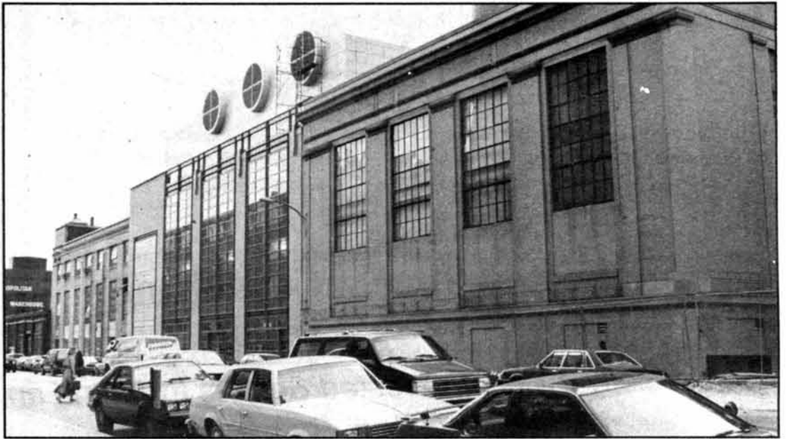
The new cogeneration power plant is at the center of a legal dispute between the state Department of Public Utilities and MIT.
