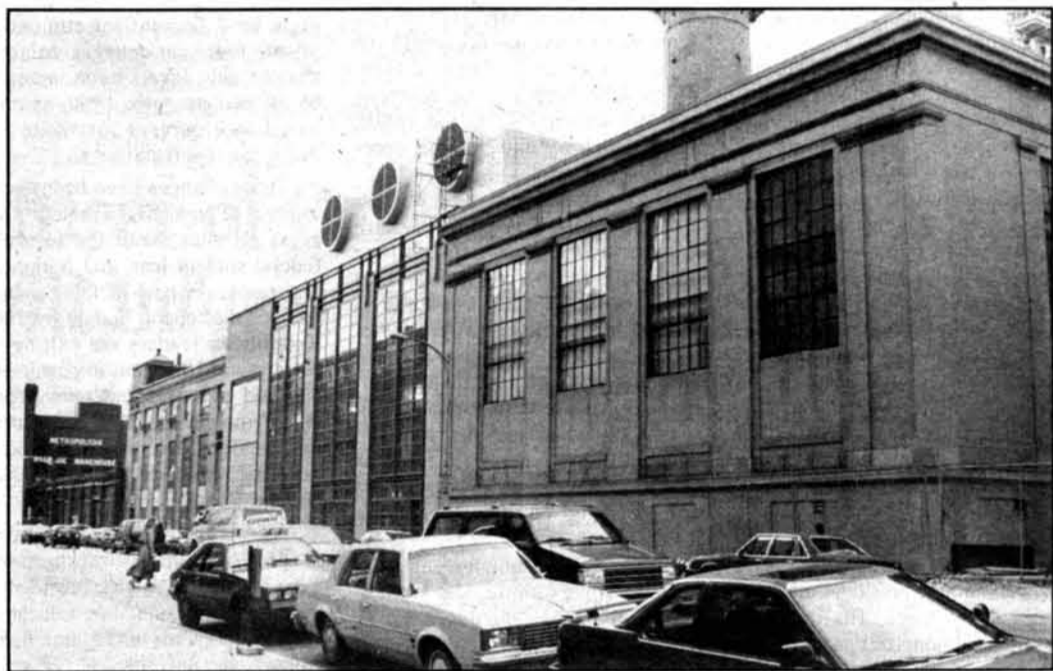
The $37-million cogeneration plant began operation Sept. 11.
