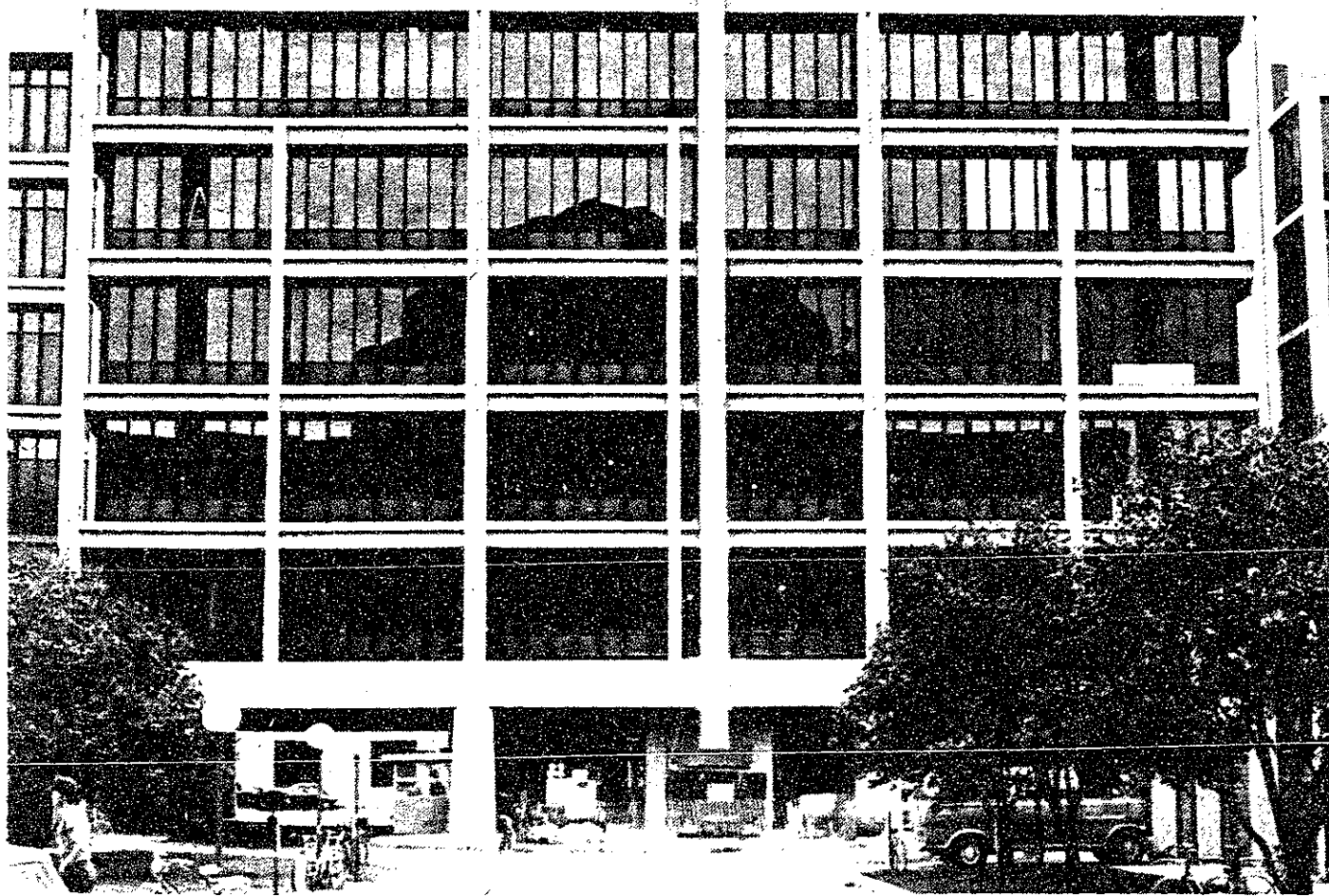
Building 39 undergoes renovation.
