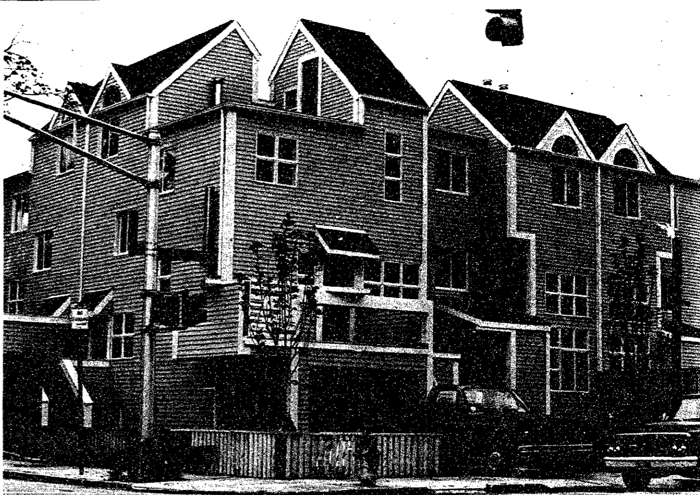
Tech Photo by Rod Wester
