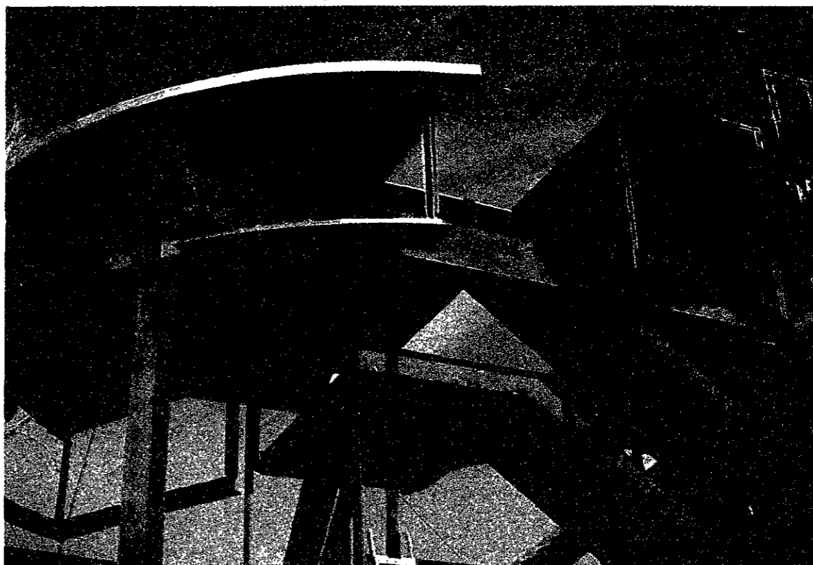
Construction continues on the ice rink - field house - events center that is scheduled to be completed by the end of this year. (Photo by Matthew B. Alschuler)
